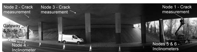
Fig. 6. Node layout at the Ferriby Road Bridge
